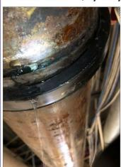
Replacing main plumbing lines at Sanfordville that are used for both heating and air conditioning throughout the building. The entry pipe and main pipes to Park Avenue, which have been repaired, now need to be replaced. These projects will cost \$1,100,000.
