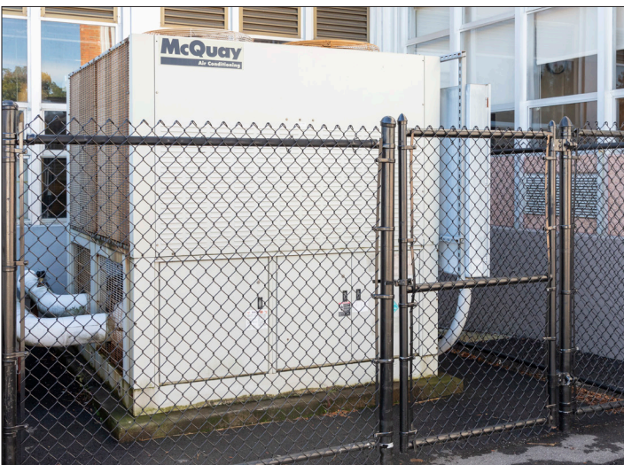
Two air conditioning chiller units at the High School are old, failing, and need to be replaced.
