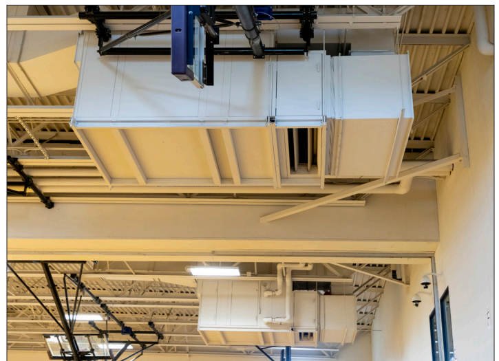
The gym unit ventilators in the Middle School and High School are ineffective and need to be replaced to create a healthier breathing environment.
