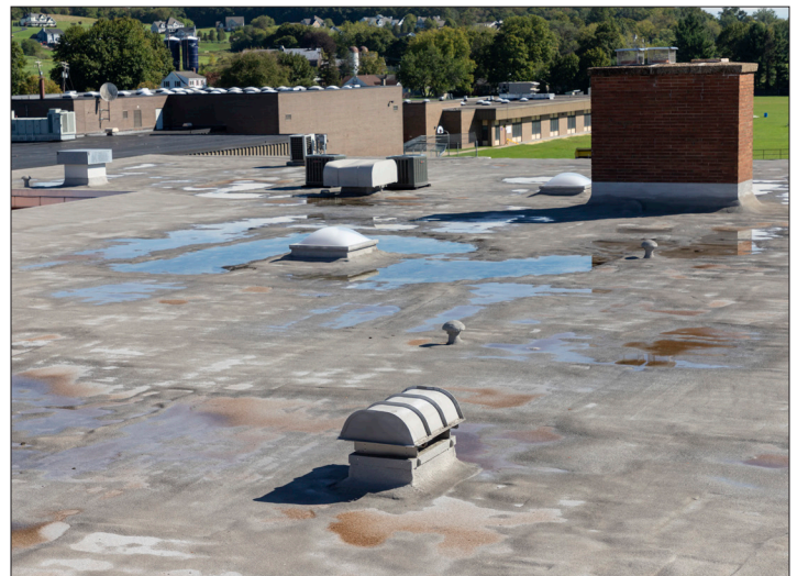
The portion of the roof at the High School made of spray foam needs to be replaced. Expansion and contraction cause cracks each season.
